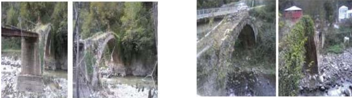
Picture 2. 13th century bridge (not restored).
