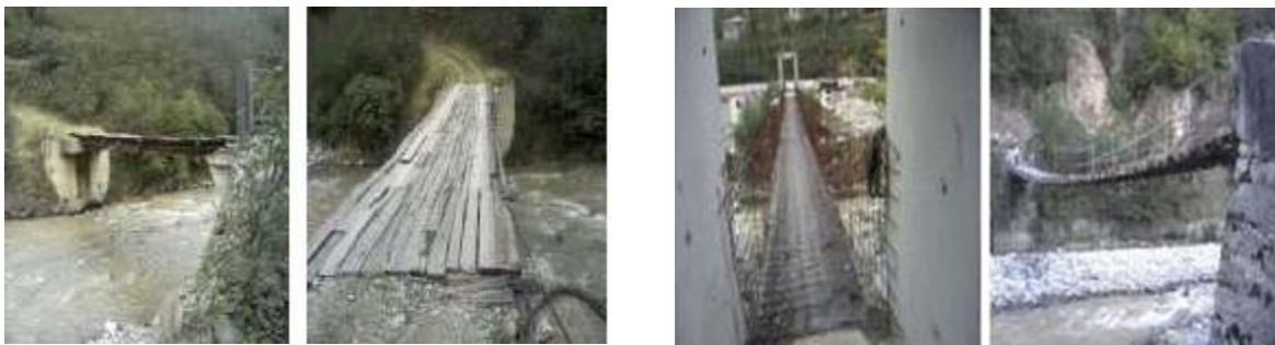
Picture 4. A 20th century suspension timber bridge.
